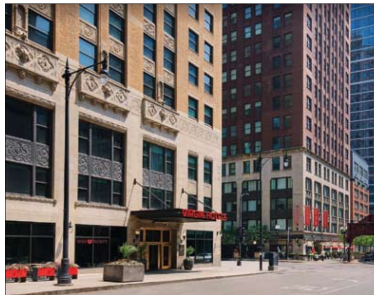
In 2015, the historic Old Dearborn Bank building was converted into a Virgin Hotel with 250 guest rooms. It is now being converted into a sports-themed timeshare property.
