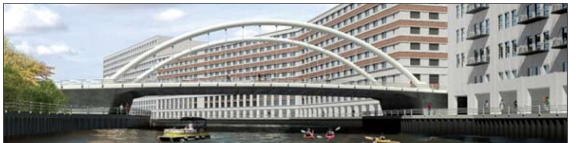
Chicago Ave. will fully close to all traffic between Larrabee and Peoria streets starting Monday, Sept. 29 for the reconstruction of the Chicago Ave. Bridge.
