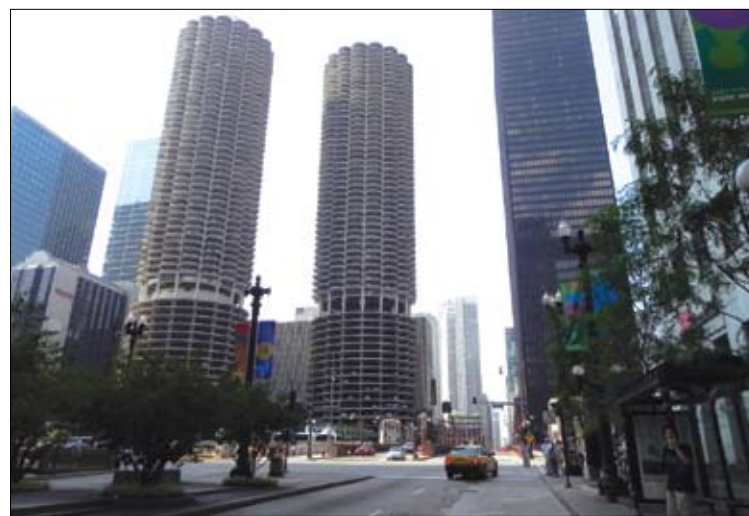
One reason for today's deconversion push is that condo resale values plummeted during the Great Recession, and prices have not fully recovered in most buildings.
