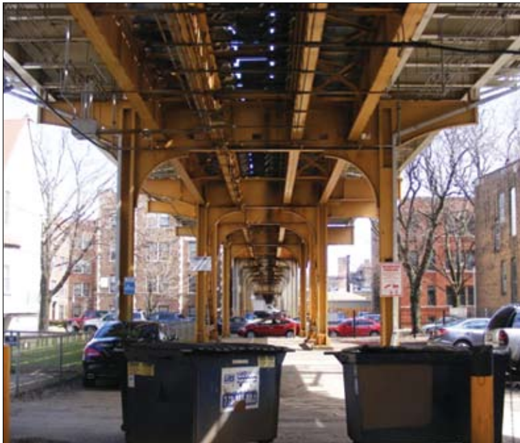
A plaza underneath the Brown Line CTA tracks between Paulina and Southport is expected to bring new life to a, noisy dark corner of Lakeview.
