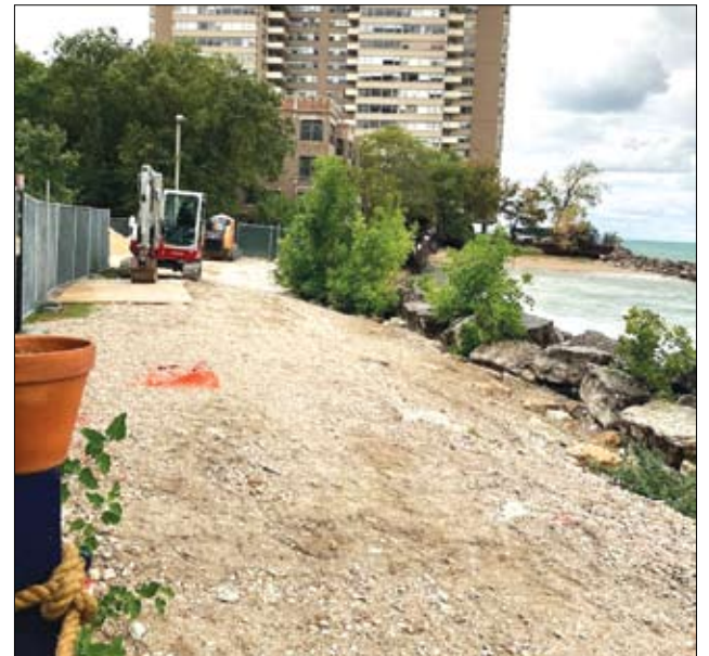
Berger Park, 6205 N. Sheridan Rd. is under construction.
