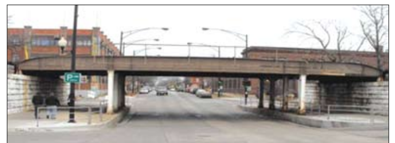
Metra bridge at Irving Park Rd.
