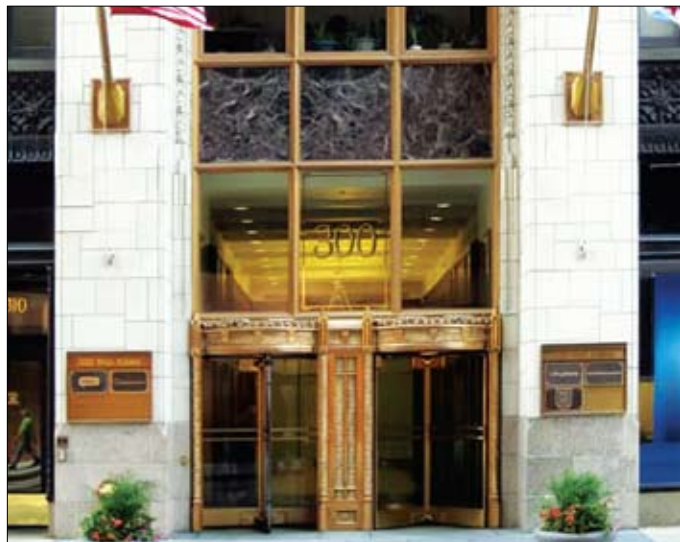
Main entrance (left) to 300 W. Adams St.
