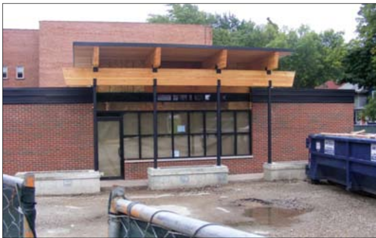
Work has already started converting the former Rogers Pantry, a former package goods liquor store at 1930 W. Chase into a medical marijuana dispensary.
