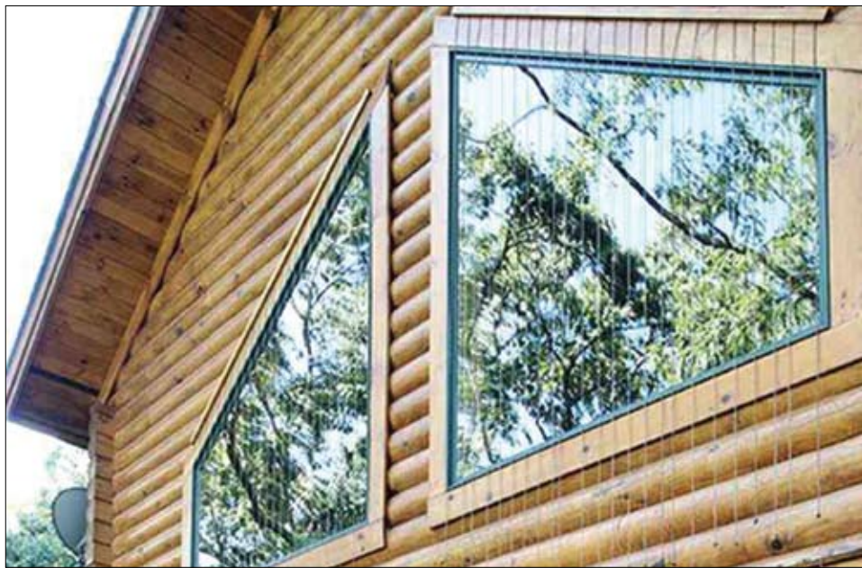
Zen wind curtains (above) designed to be installed on the outside of the glass are made from paracord and can be custom-fitted to your windows. Photo courtesy of Dr. Ellen K. Rudolph
