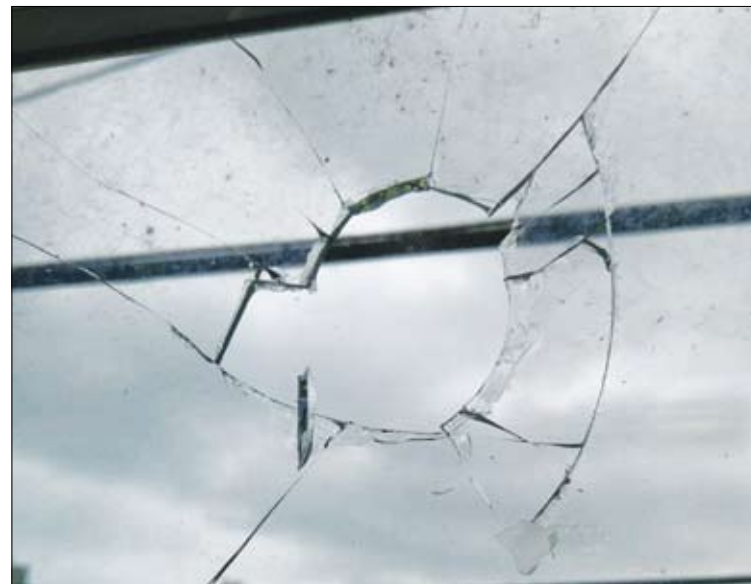
The window of Inside Publication's headquarters was broken by a thrown rock at 3 a.m. on Sept. 22.
