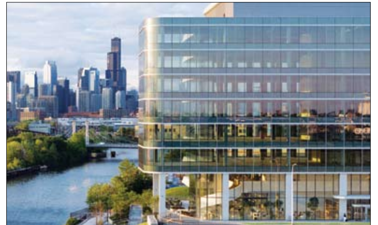
The vacant Life Science building at the former Lincoln Yards development, which is now called "Foundry Park."
