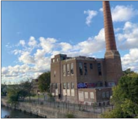
The Lathrop Homes powerhouse.
