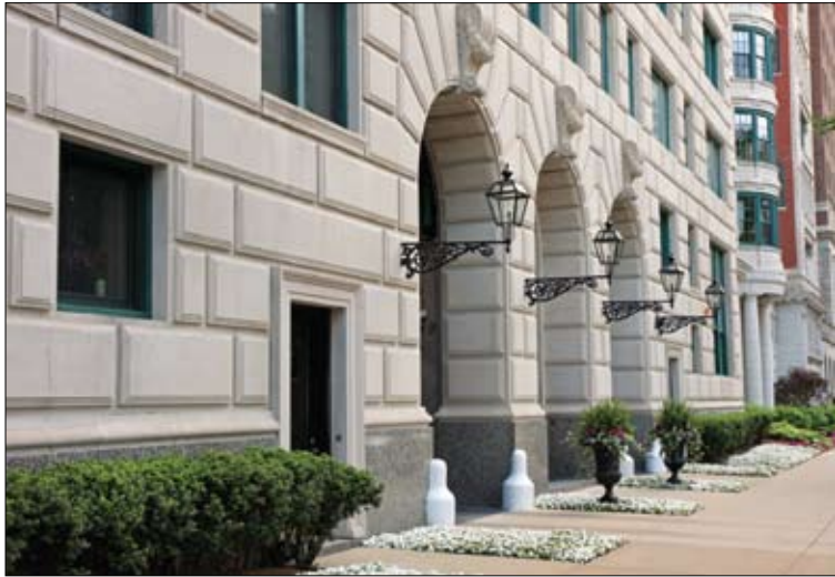
Benjamin H. Marshall (1874-1944) had a major impact on Chicago architecture, and now will have a street dedicated in his honor. Pictured above is the Marshall-designed 209 E. Lake Shore Drive.
