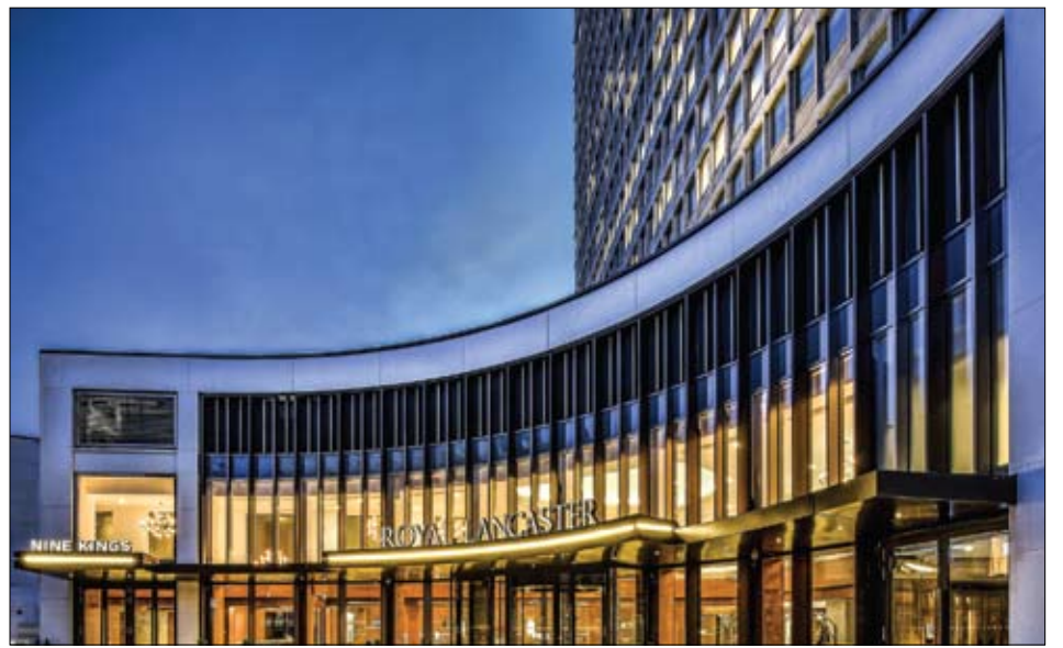
The Royal Lancaster London, which overlooks Hyde Park and Kensington Gardens, has been completely transformed both internally and externally.
