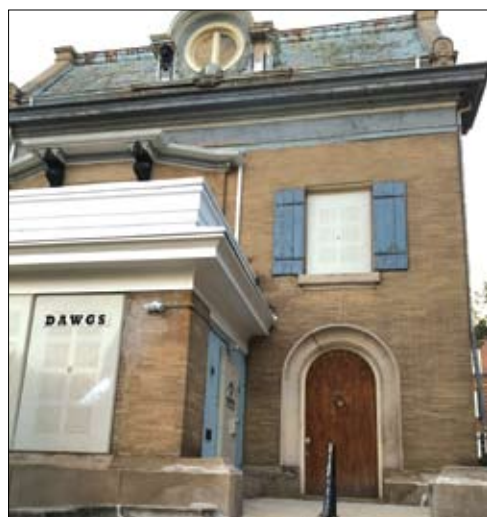
This boarded-up 19th century mansion at 4506 N. Sheridan Rd. once house the Neon Street Dorm.
