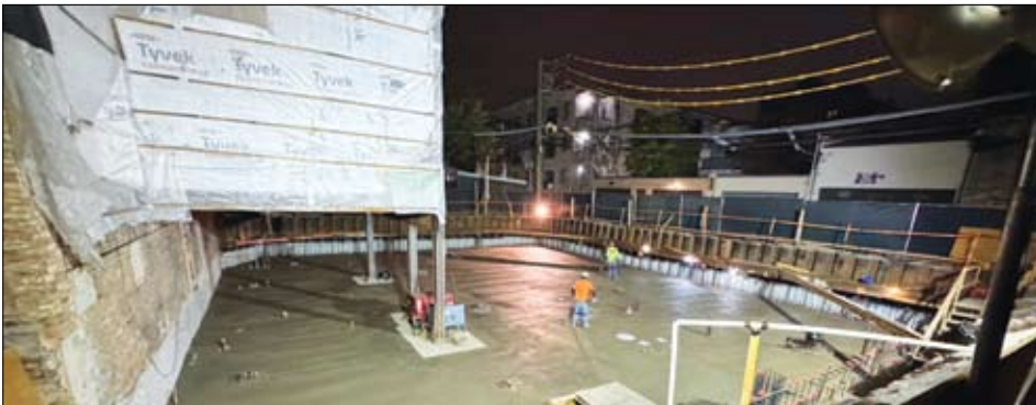
The Care For Friends charity is moving swiftly constructing their new homeless shelter in Lincoln Park, and last week their construction crew poured 12 inches of reinforced concrete as a foundation for their new space at 530 W. Fullerton.
