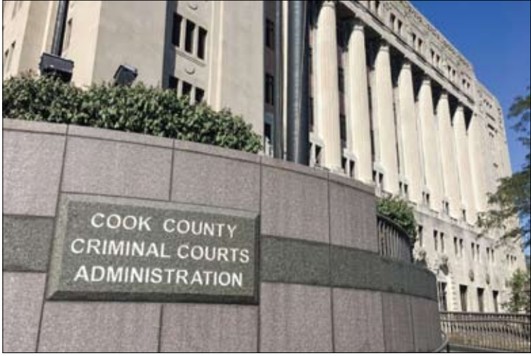
The Cook County Criminal Courts Administration Building, 2650 S. California Ave., next to the George N. Leighton Criminal Court Building in Chicago. Photo courtesy of Erica Snow
