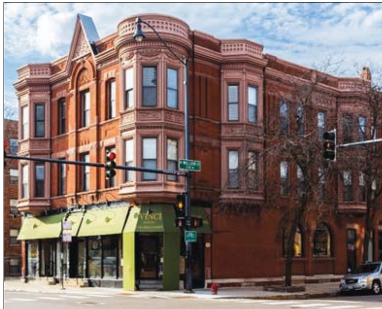
1730-1732 N. Halsted St. Courtesy City of Chicago Dept. of Planning and Development
