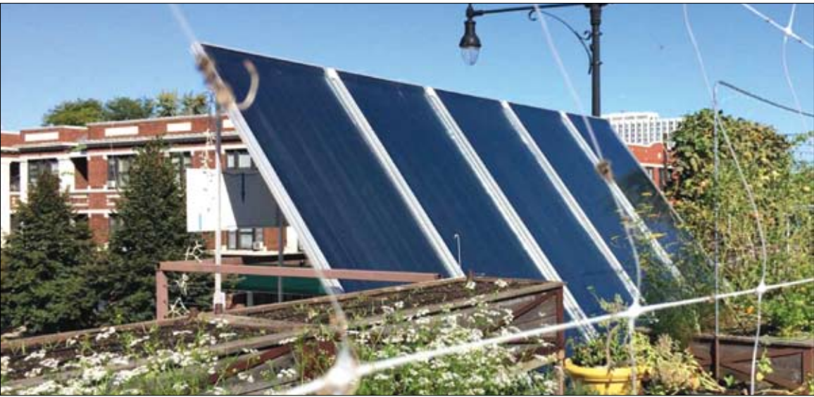
Uncommon Ground’s five solar thermal panels on the restaurant’s rooftop farm provide about 10% of its overall energy needs.
