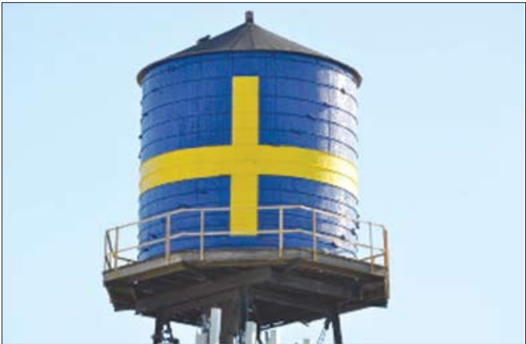
The Andersonville Water Tower Tank that was perched on its roof for almost nine decades.
