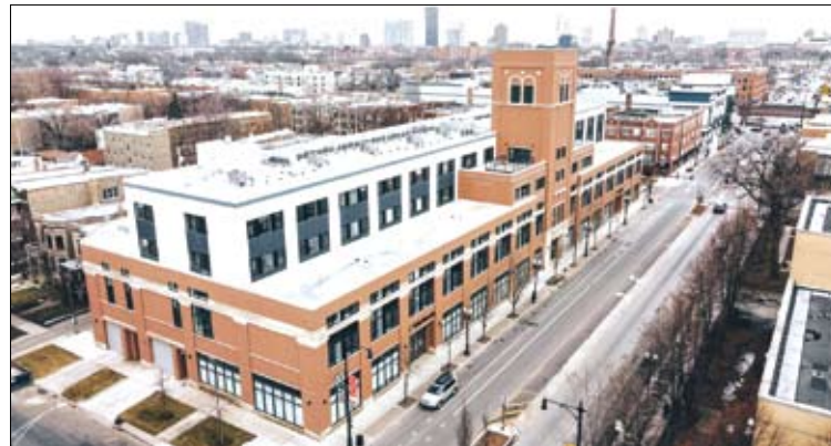
The mixed use building at 1900 W. Lawrence Ave. was built to be a Sears Department Store.
