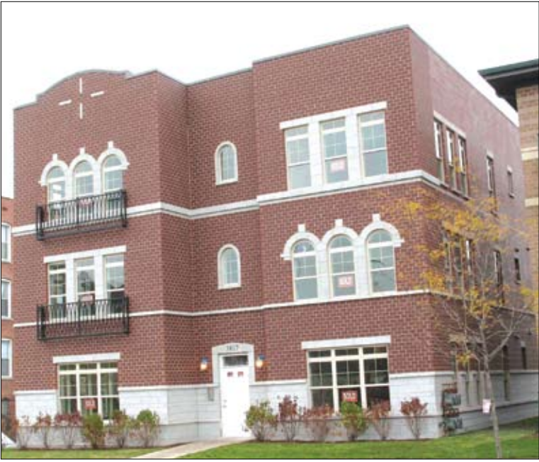
A new six-flat in the Oakwood Shores development in the Oakland/North Kenwood neighborhood.
