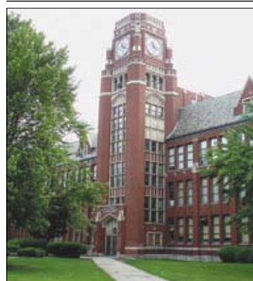
For over 15 years, the aging clocks in the clock tower have not worked.
