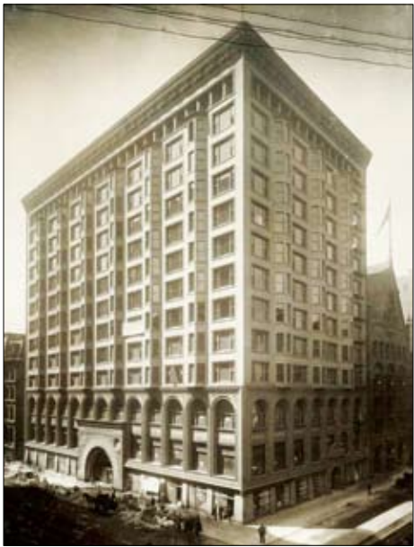
The former Chicago Stock Exchange building, famously demolished in 1972.
