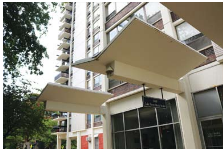
Carl Sandburg Village, 1355 N. Sandburg Terrace.
