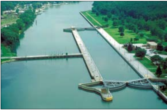
T. J. O'Brien Lock and Dam on the Calumet River, part of the Illinois Waterway that includes the Chicago River. Photo by Carol Arney, U. S. Army Corps of Engineers.
