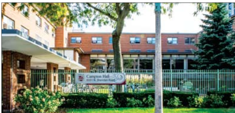
Campion Hall at 6551 N. Sheridan will fall under the wrecking ball in May of 2025 to pave the way for a new academic building. Constructed in 1955, Campion Hall was the first residence hall at Loyola and the first on the Lake Shore Campus. Photo courtesy Loyola Univ.
