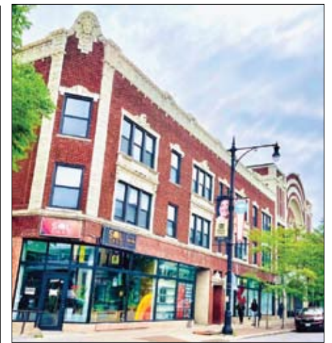
In 1999, the long-vacant Howard Theatre's auditorium was razed but its beautiful façade and outer lobby were saved and integrated into the apartments and retail structure which was built on the site.
