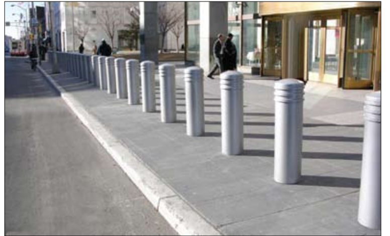
Concrete bollards are sturdy vertical posts installed to protect buildings, guide traffic, and act as pedestrian safety barriers.
