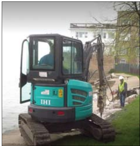
Work is underway at Juneway Beach on much-needed revetment repairs.
