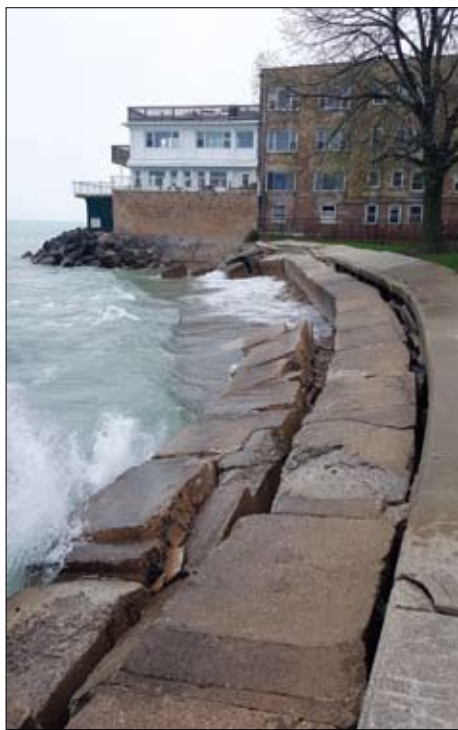
The eroded revetment at Juneway Beach.
