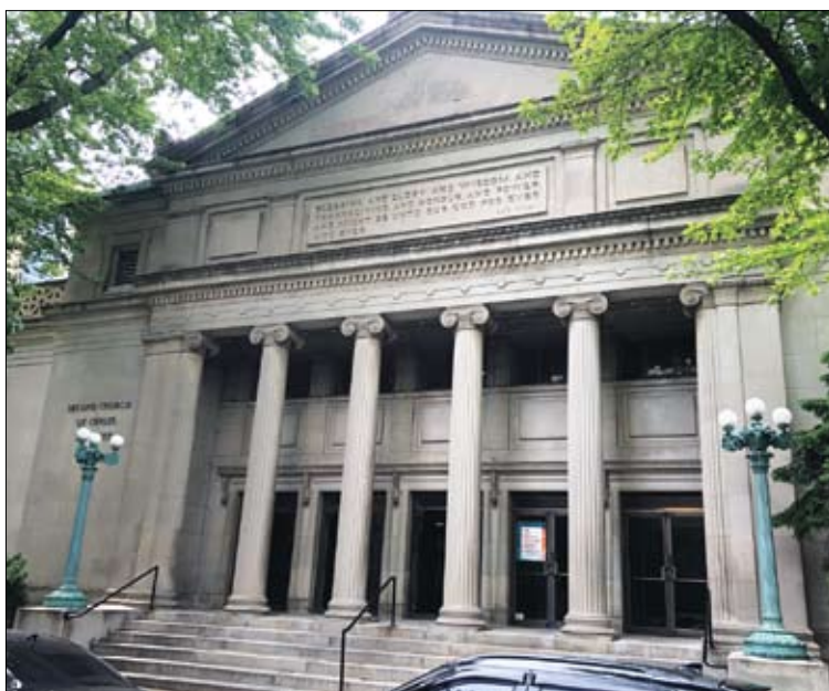
The 2nd Church of Christ Scientist building at 2700-27017 N. Pine Grove Ave. in Lincoln Park will soon be under construction, with a new 6-story mid-rise added to the site.
