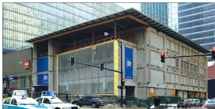
(Top) Actor John Mahoney, longtime broadcaster Hugh Downs, museum president Bruce DuMont, and actress Betty White cut the ribbon to officially open the Museum of Broadcast Communications on June 13, 2012. (Bottom) State and Kinzie, during the construction phase, on December 18, 2008.
