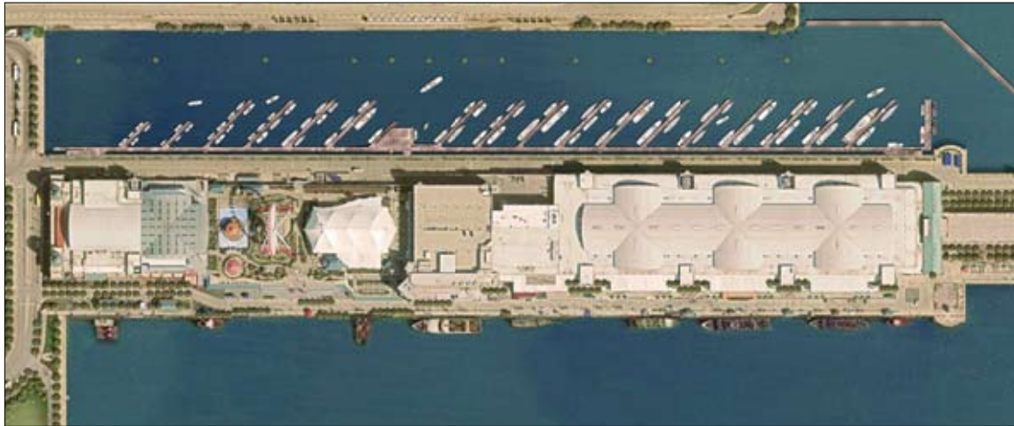
Navy Pier will soon start construction on the newest transient boating destination on Lake Michigan, their new all-transient marina.
